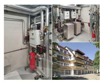
freshwater modules are regulated and controlled by means of an ApacoLogic control system, which was designed and built on a plant-by-plant basis in APACO's automation department. The creation of this modern freshwater station was accompanied by the APACO team by means of a comprehensive service package.
