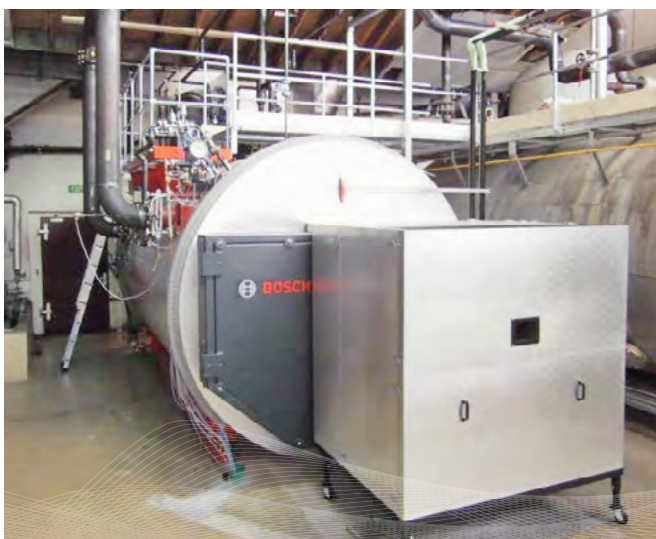
| UL-S steam boiler with an output of 5300 kW
