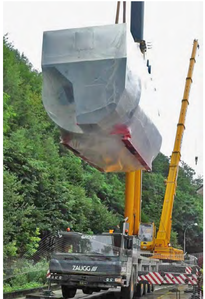
| Placing the boiler in the boiler house
